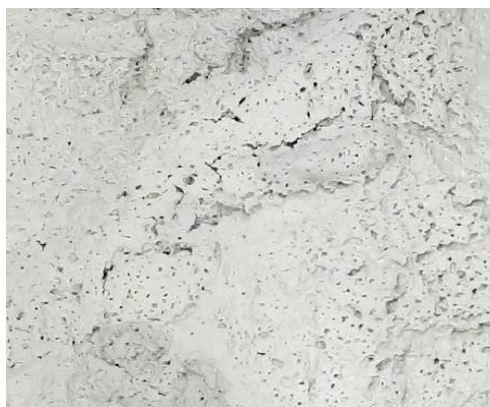
AFTER PARTIAL DRAINING
