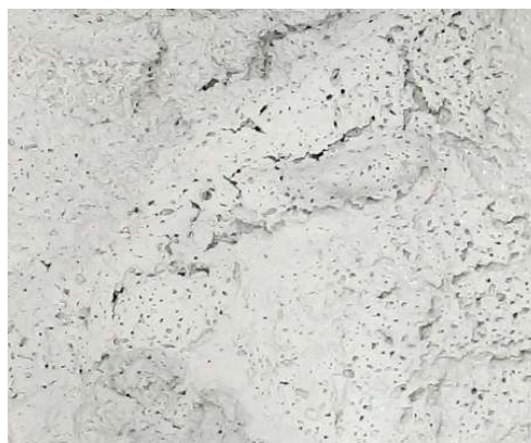
AFTER PARTIAL DRAINING
